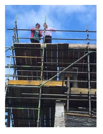
The work involved erection of scaffolding to provide a safe working platform, raking out of old broken material and re-pointing with lime mortar. Other works carried out included the replacement of bell carriage support timbers, painting of the bell carriage and renewal of bell pull chains and linkages.
